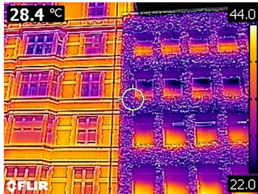
Figure 15. Infra-red image of masonry wall (left) and green wall (right).
